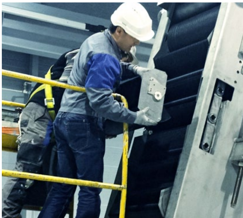
Filter element can be dismantled from the front
